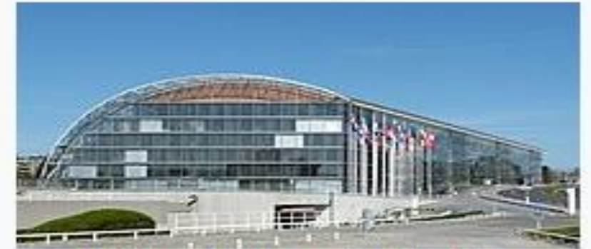
EIB headquarters, East building
