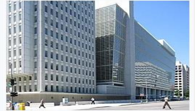
The World Bank Group building in Washington, D.C.
