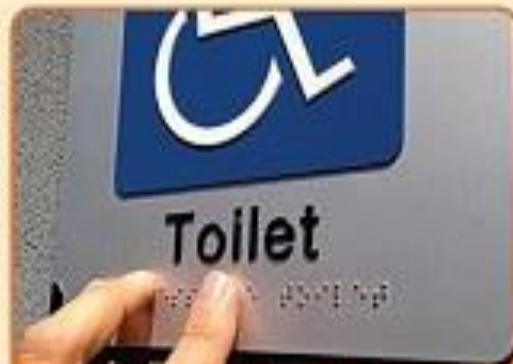
Braille Signage for Visually Impaired
