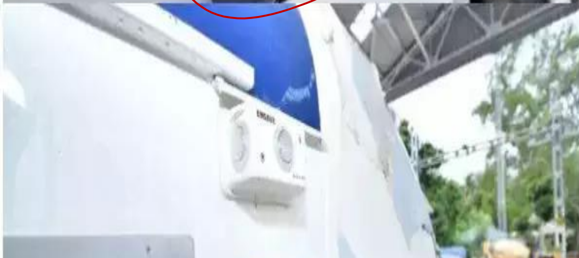
New platform side cameras and signal exchange lights
